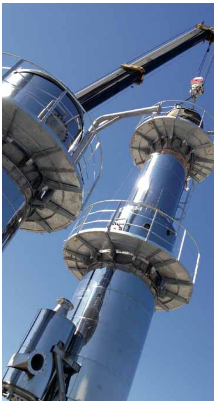
The plant is now operating at 100% capacity
